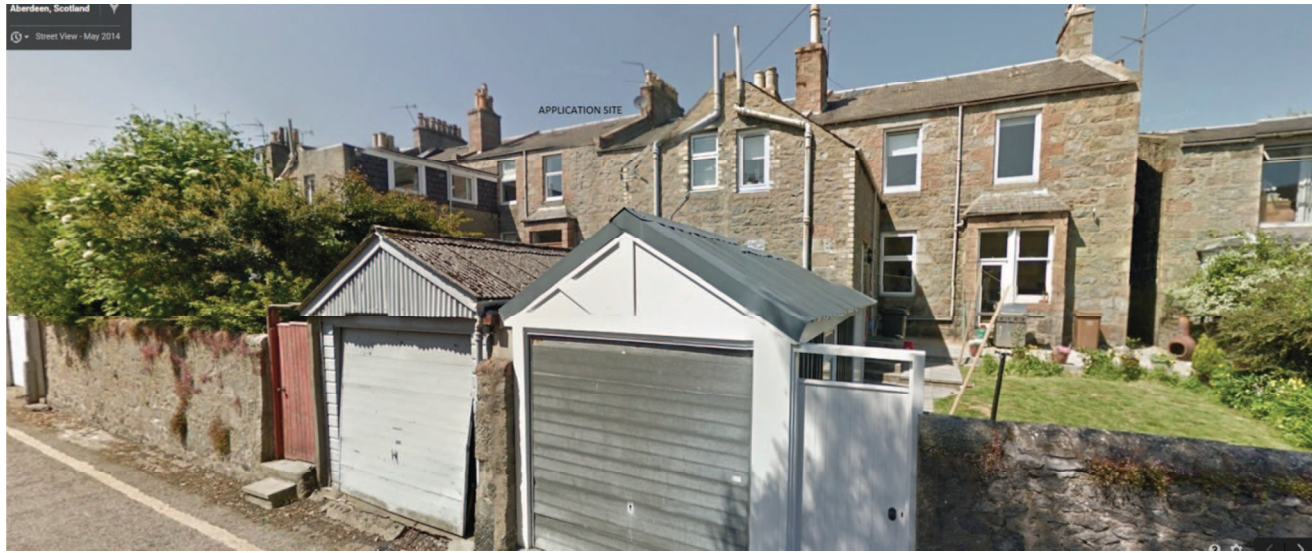
View of site from rear service lane. Note the prominence of modern garages, alterations to rear wing of application site, chimney stacks half way down the roof & existing large box dormer at no 43.
