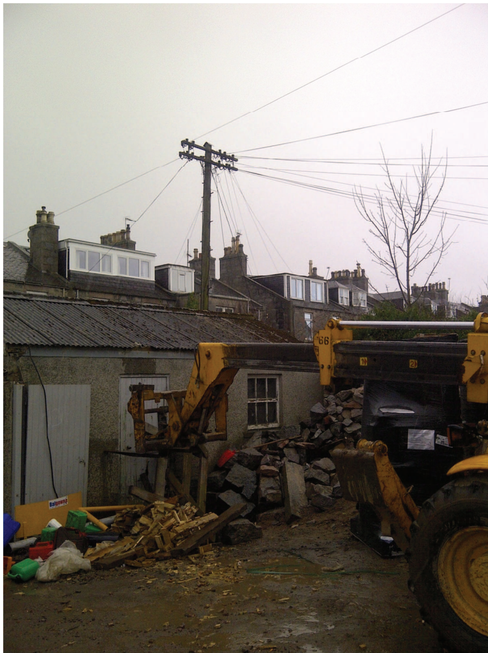
Picture above of a recently approved Dormer at 6 Carlton Place (Ref: 121229). Note large slate apron, closer projection to tabling and further forward projection.
