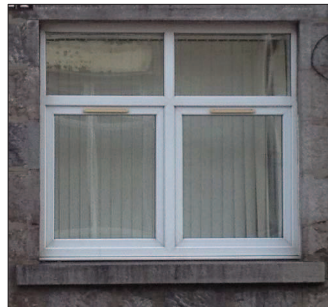
Discreet means of achieving ventilation will be required for Listed Buildings and on public elevations in Conservation Areas
