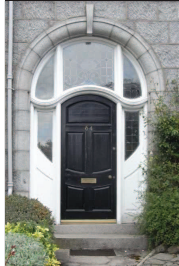
Windows, doors and doorways can be important features of a building which are important to protect
